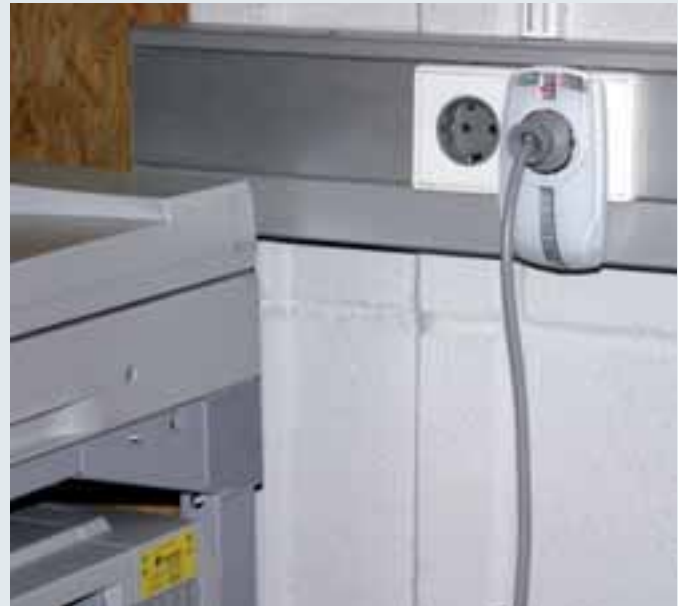
Adapters for protecting the power supply of electronic devices against the effects of transient surges as well as high-frequency interference voltages (DEHNpro 230 F Protector)
