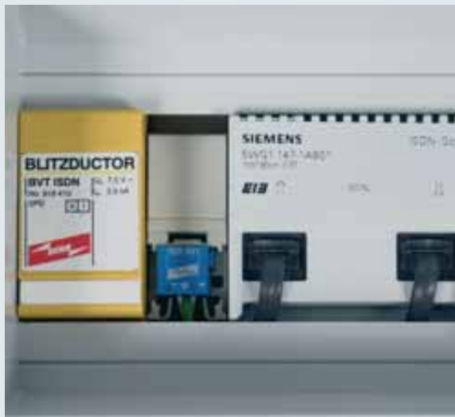
Surge arrester for EIB / KNX buses with connecting leads.
