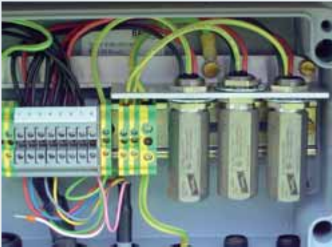
Surge arrester for outdoor use for screwing into 2-conductor process field devices. Stainless steel. Allows for installation up to IP 67.
