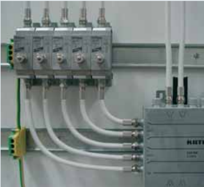
Lightning current and surge arrester for use as a cable adapter for coaxial systems such as CCTV, cell sites and antenna systems.
