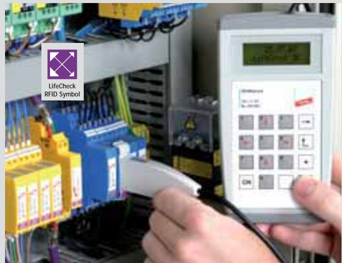
Testing an SPD module for use in intrinsically safe circuits (blue-coloured) by means of RFID technology (LifeCheck)
