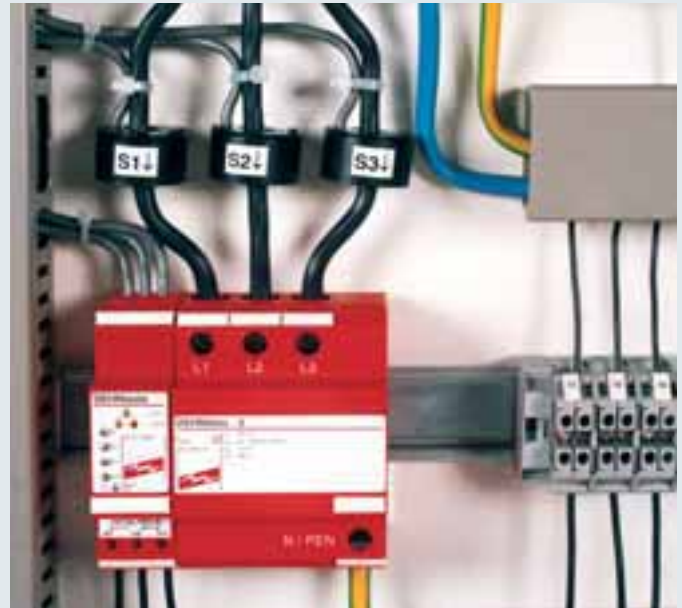
Continuous function test of installed lightning current and surge arresters by DEHNisola monitoring device.
