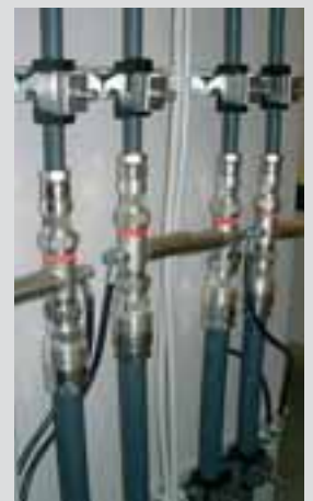
Application of Lambda/4 arresters
