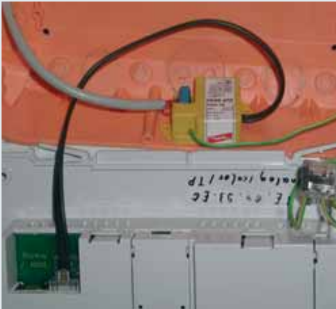
Surge arrester for flush mounting used in LAN interfaces.
