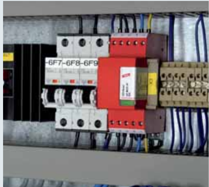
For protecting the power supply of industrial electronic devices in switchgear cabinets against surges.
