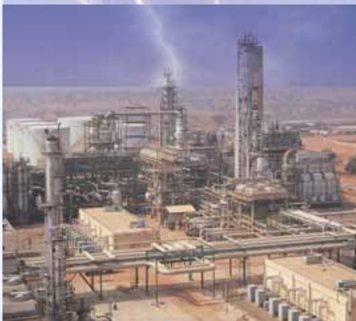
Process technology – safely protected by DEHN!
