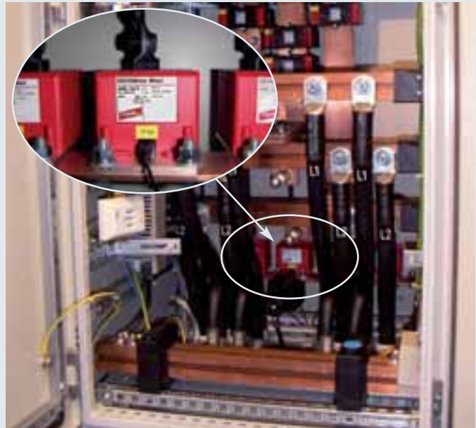
For protecting low voltage consumer's installations against surges. For use according to the lightning protection zones concept at boundaries 0_A - 1 .
